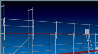
Now, the next level can be safely fitted with the help of the securing guardrail. Subsequently, the guardrail again moves upwards.
