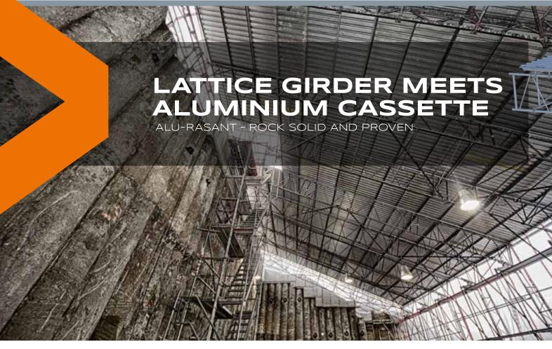
Although on the market for some time now, it is still our most successful roof and wall system. Building sites can be optimally covered with the combination out of lattice girders, roof cassettes and bracing elements. Span widths of up to 40 m can be easily accomplished.
